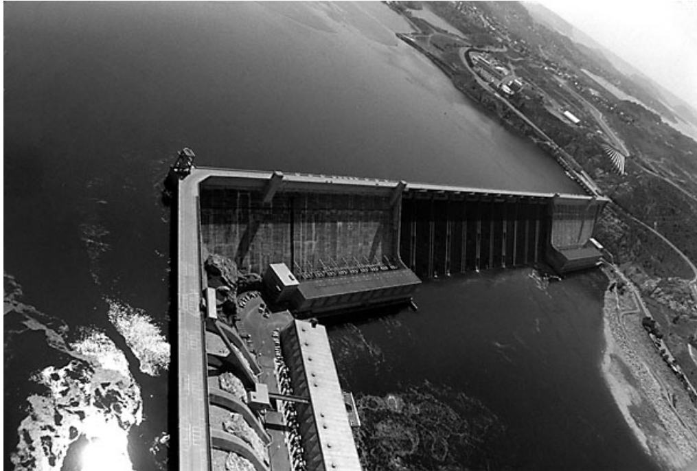
Aerial view of Grand Coulee Dam with Powerhouse 3 in the foreground
